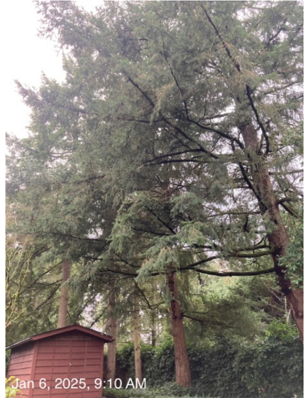
Trees #21-#25 noted as healthy and vigorous. Shed foundation damage noted caused by soil displacement from root growth.
